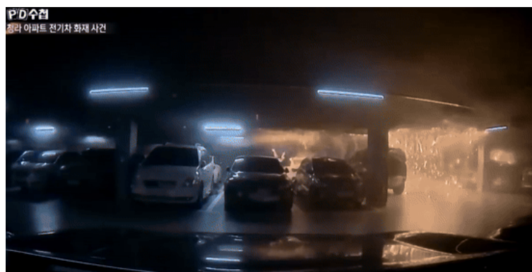
FIGURE 18 IMAGE FROM DASHCAM FOOTAGE SHOWING IGNITION OF CEILING PRODUCTS IN THE INCHEON CARPARK FIRE SOON AFTER THE FIRE BROKE OUT (SOURCE: NEWS 1 KOREA 2024 98 )
